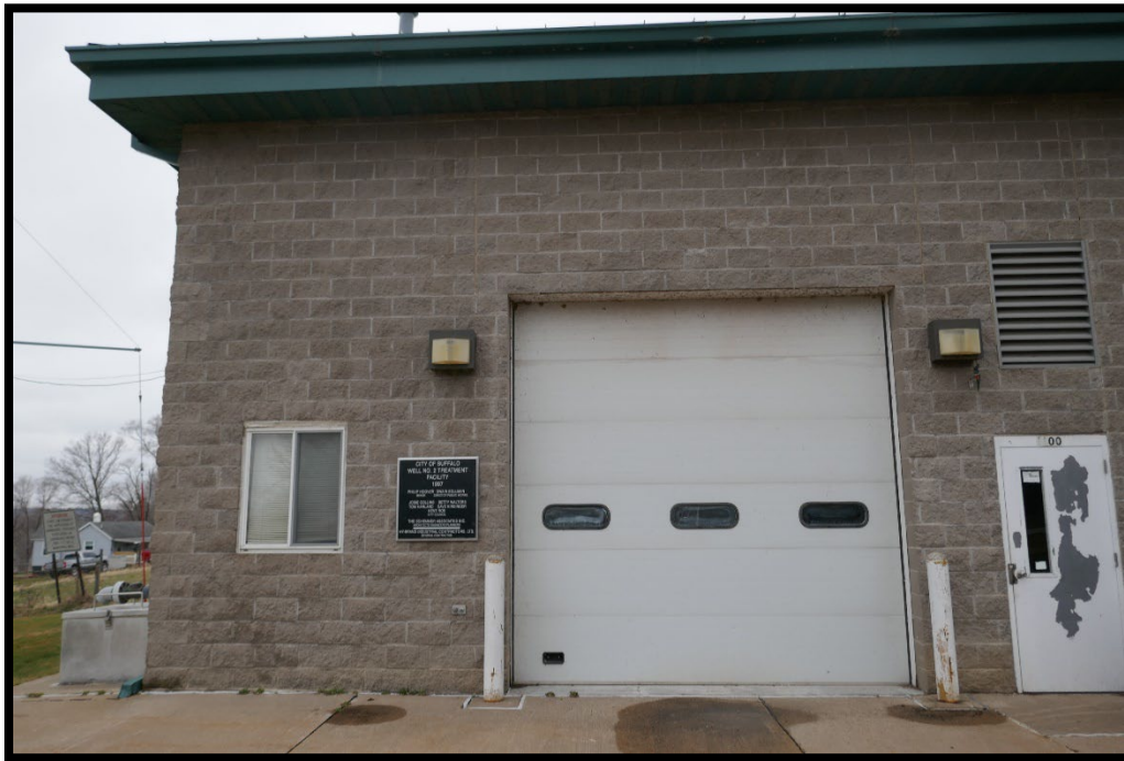
Water Treatment Plant
