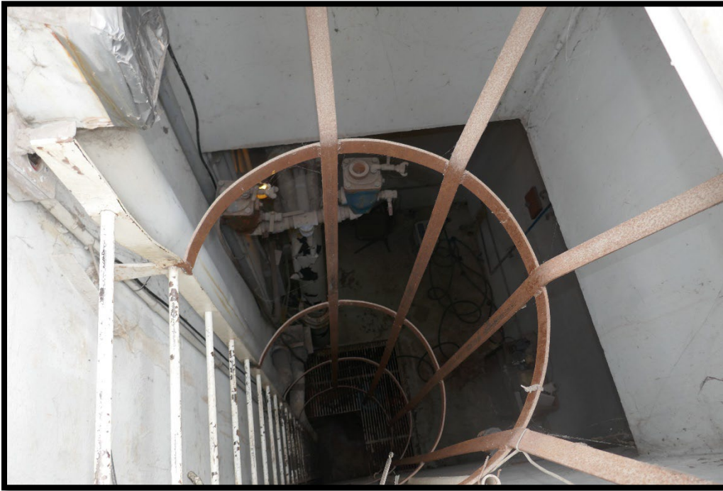
Interior – East Lift Station
