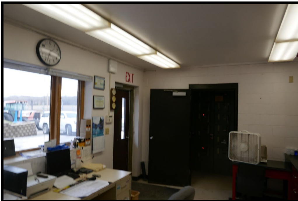
Interior - Wastewater Plant
