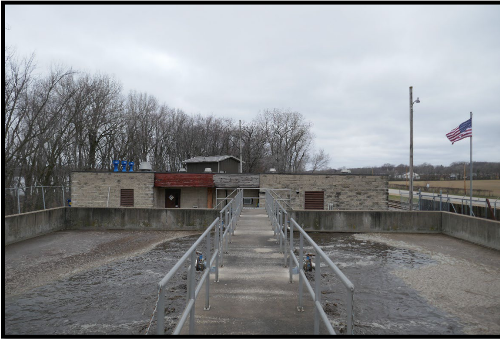
Wastewater System and Wastewater Plant
